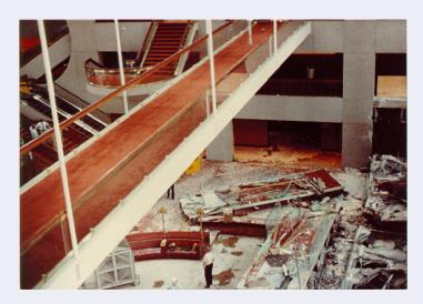
Design flaws were found to be the cause of the collapse. The third-floor bridge did not collapse but was later removed. Only the current, second floor bridge was rebuilt.
